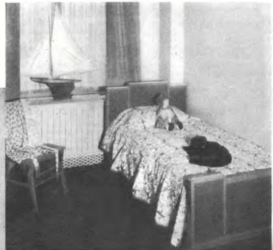
2—One of the new radiators built into a window
