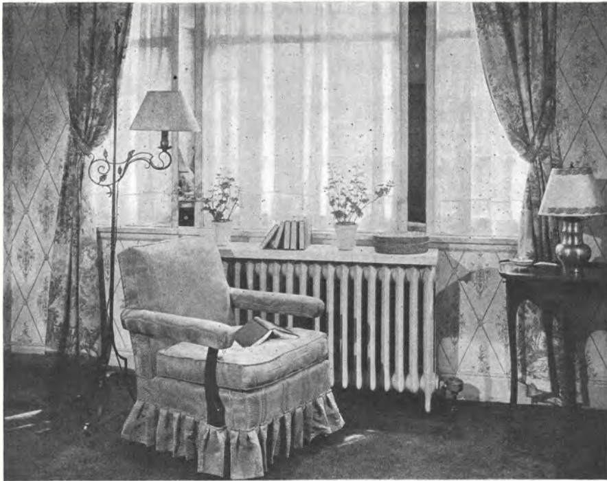
1—A covered radiator has four advantages: it is economical of steam; looks better; supplies a convenient table top; and protects the window curtains from rising dust
